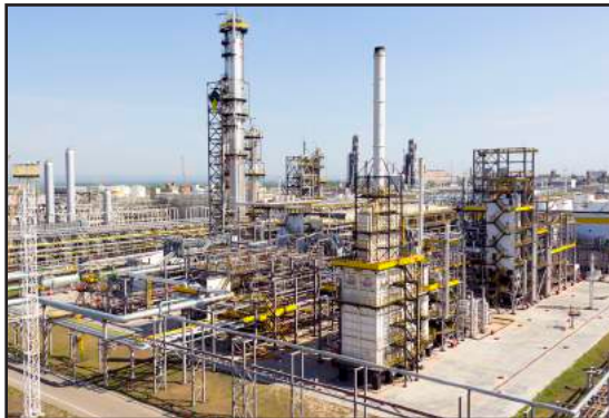
The heat exchanger operated at pressure of 20 bar (790 psi); 220°C (428°F)
