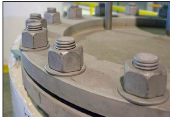
The new system provided constant pressure for the M20 bolts.
